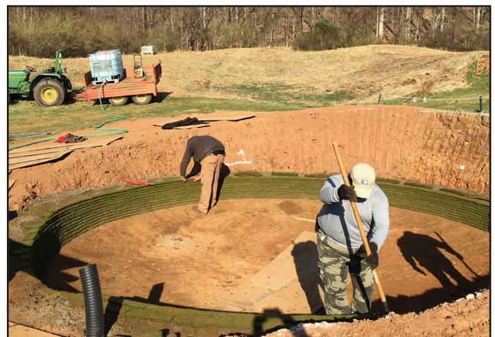
The target bunkers were medium-sized but quite deep at roughly 5.5 feet high on the high side. Bunker entry points were low, with a planned step down of 10 inches after the addition of sand.
