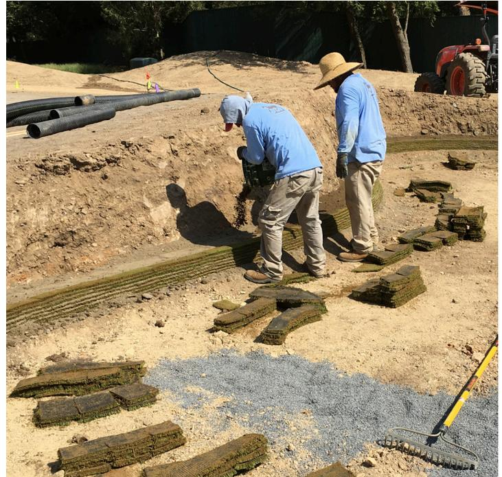
In addition to the synthetic turf spec, defined methods and materials are used to build the wall, insuring stability and durability while delivering unmatched realism and aesthetics. When assembling the PermaEdge wall, the edge of the turf is exposed. This gives bunkers an extremely natural look while the synthetic materials prevent decomposition.
